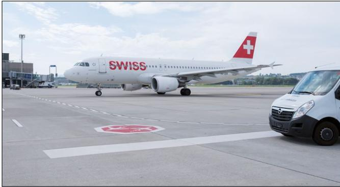
Staggered lines along the edge of a roadway indicate that it is crossing a taxiway at this point. Never stop on a roadway where it crosses a taxiway (like on a railway level crossing).
