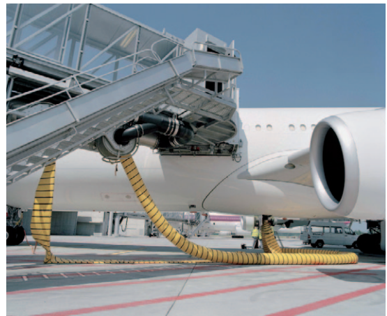
Fig. 6: Fixed Ground Power at Piers.
