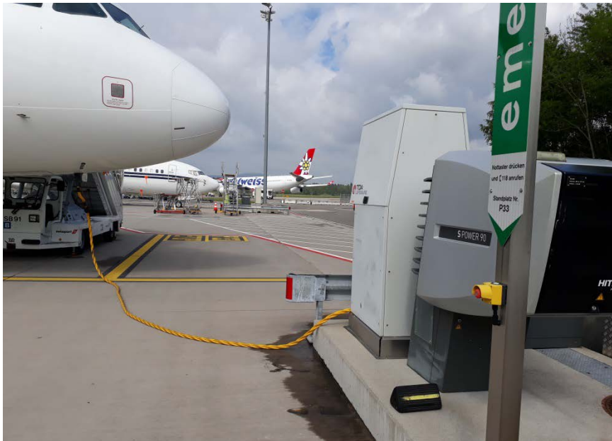
Figure 12 400Hz system open stands "Papa" Eastern Part.
