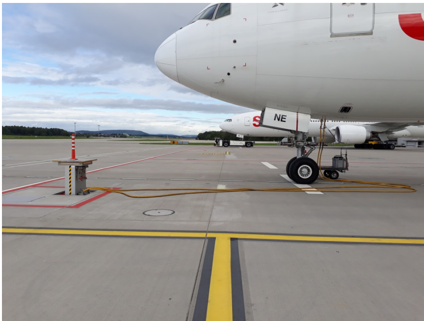
Figure 13 400Hz pit system open stands "Papa" Western Part.
