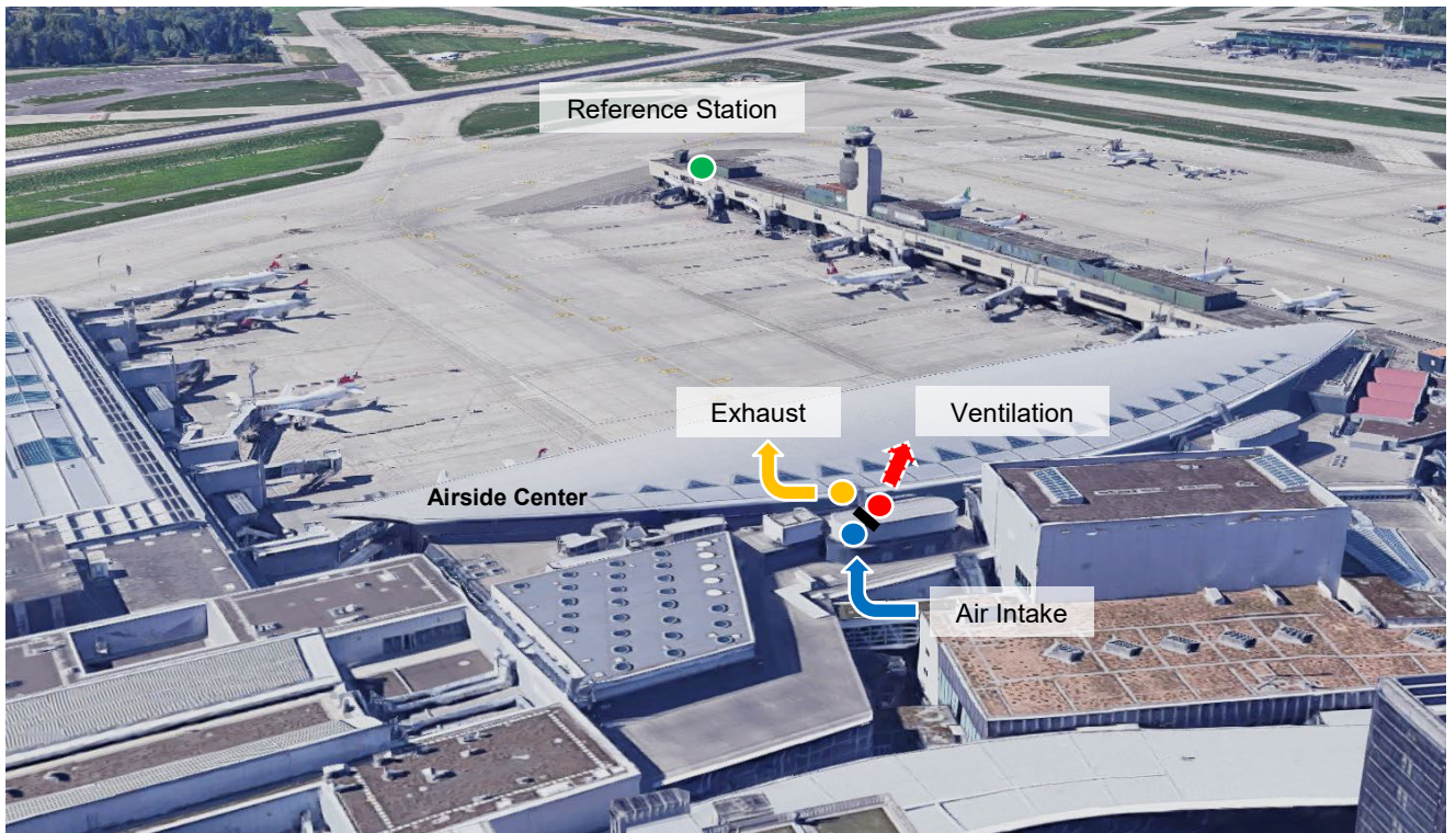
Figure 1 Situation of the Airside Center at Zurich Airport
